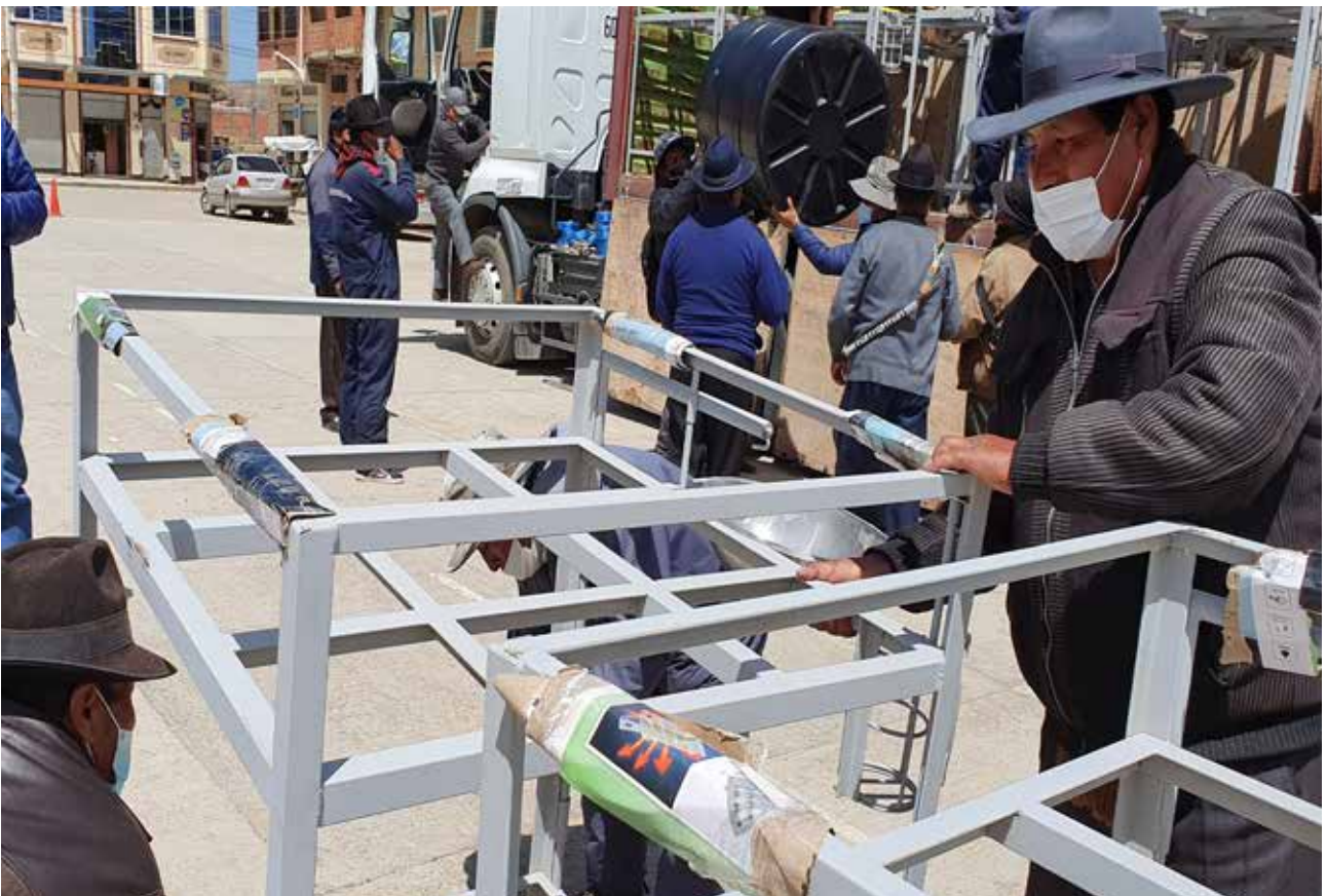
Assembly of portable hand basin, municipality of Escoma, Bolivia.
